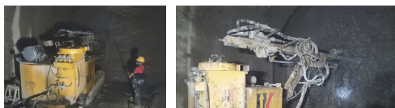
图 10 现场掌子面钻孔试验 Fig.10 Field drilling test of tunnel face
