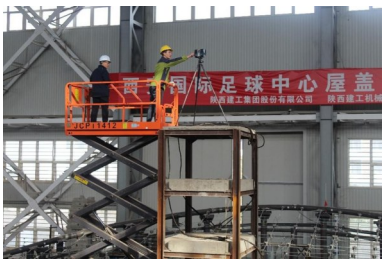
图 13 测量设备安装 Fig. 13 Installation of measuring equipment
