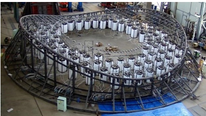
图 9 现场安装完成后 Fig. 9 On-site photo after installation completion
